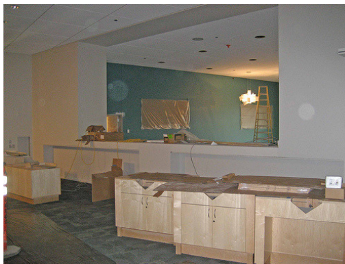
Photo of the Mastodon case under construction.
